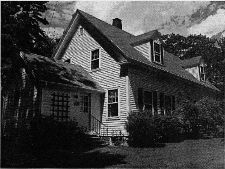
The school built in 1896 and now used for a house.
